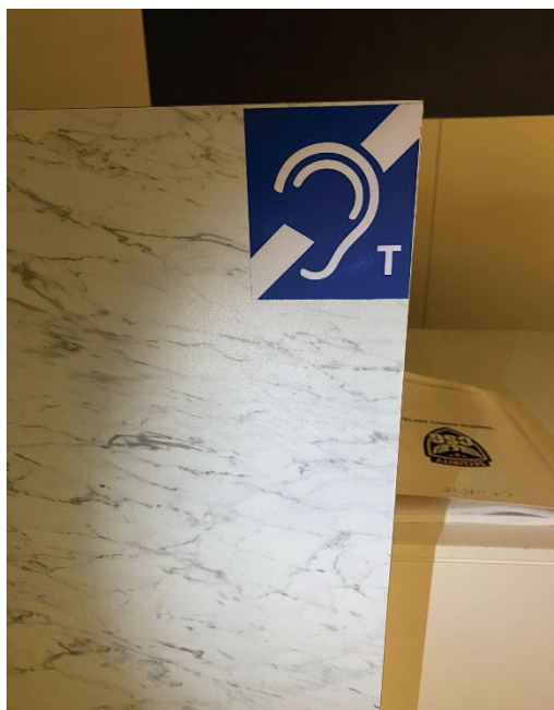
Photo 8: The hall / desk type induction loop system for disabled people.
